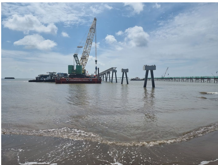
Link Bridge U-beam installation
