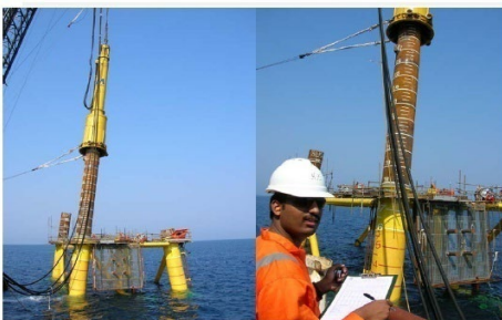
Driving of Pile with Hydraulic Hammer
