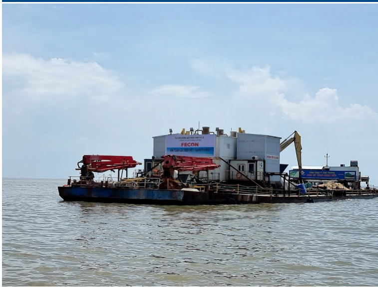
Floating batching plant-Concreting work
