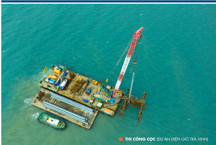
Test piling work
