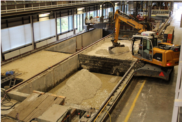
Filling tank with excavator
