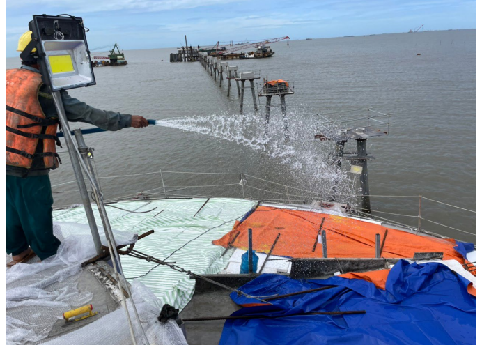
Curing concrete surface (covered by wetted jute bags and watered daily)
