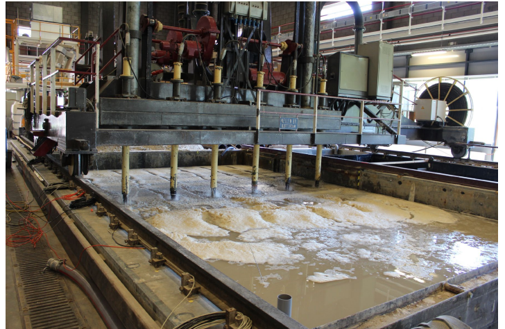
Compaction with vibrating needles
