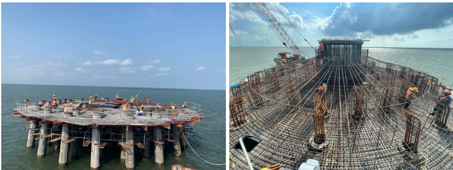
Formwork and rebar work
